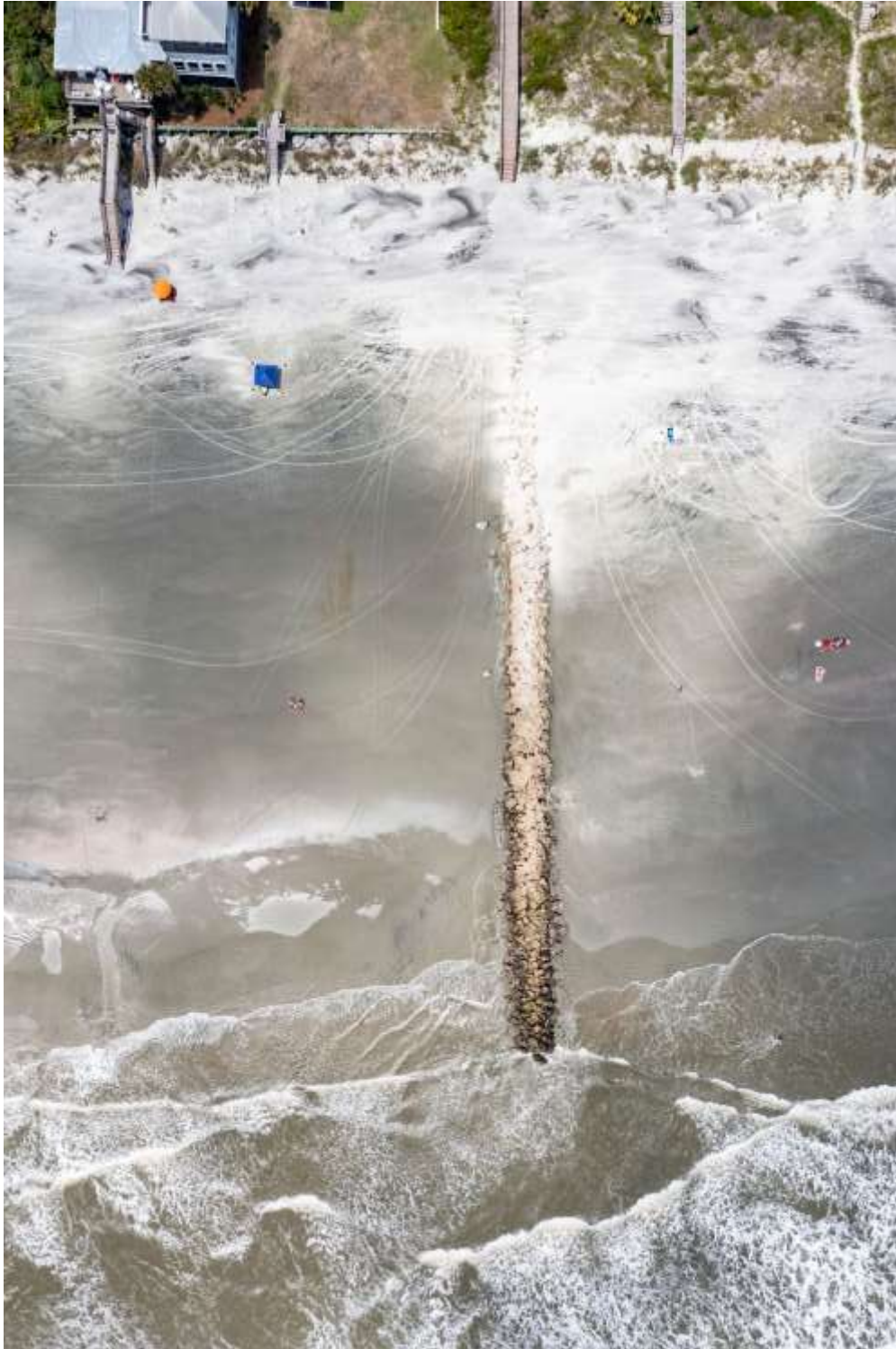
Figure 7. Groin 24 in June 2021.
