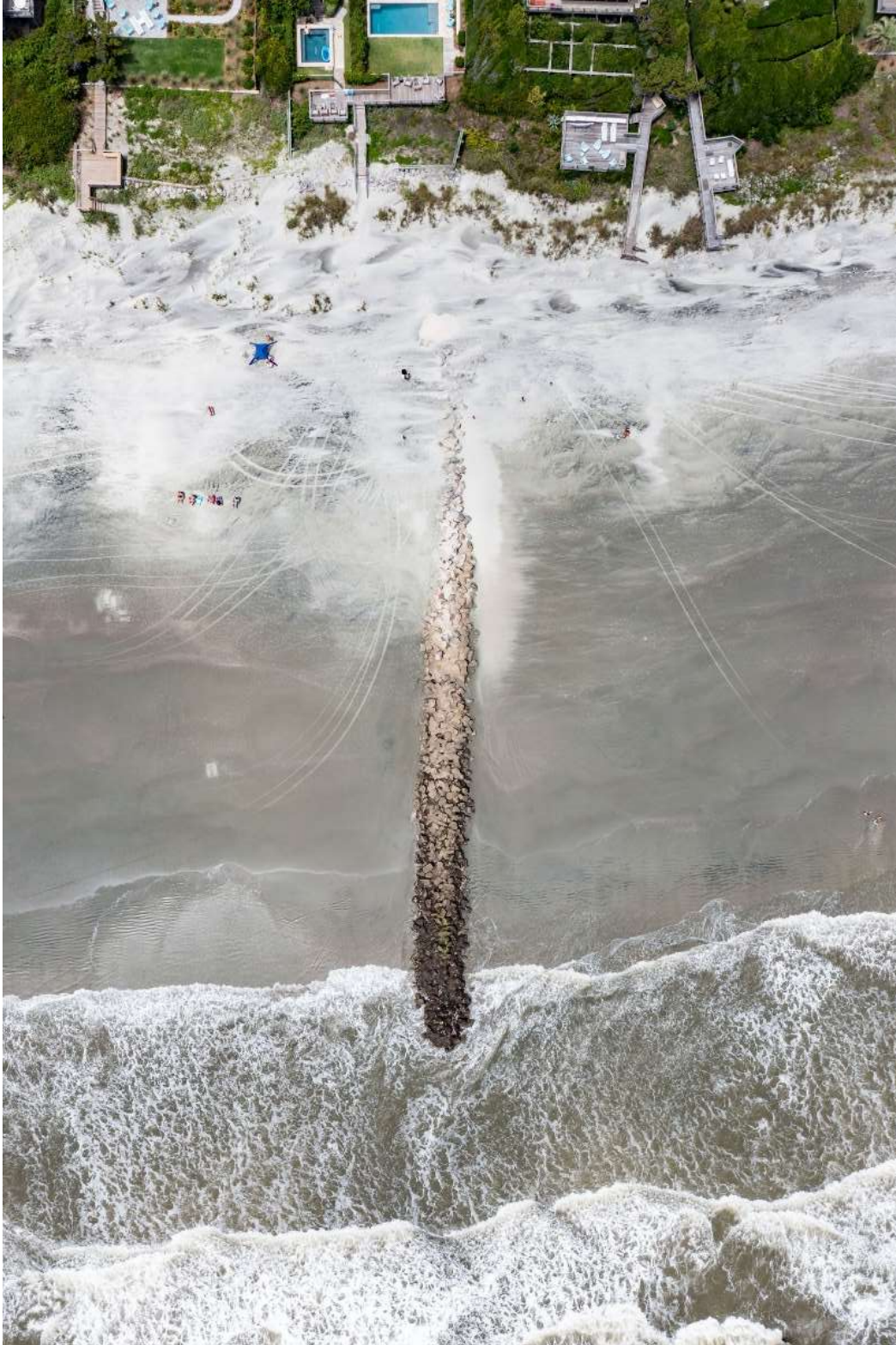
Figure 5. Groin 22 in June 2021
