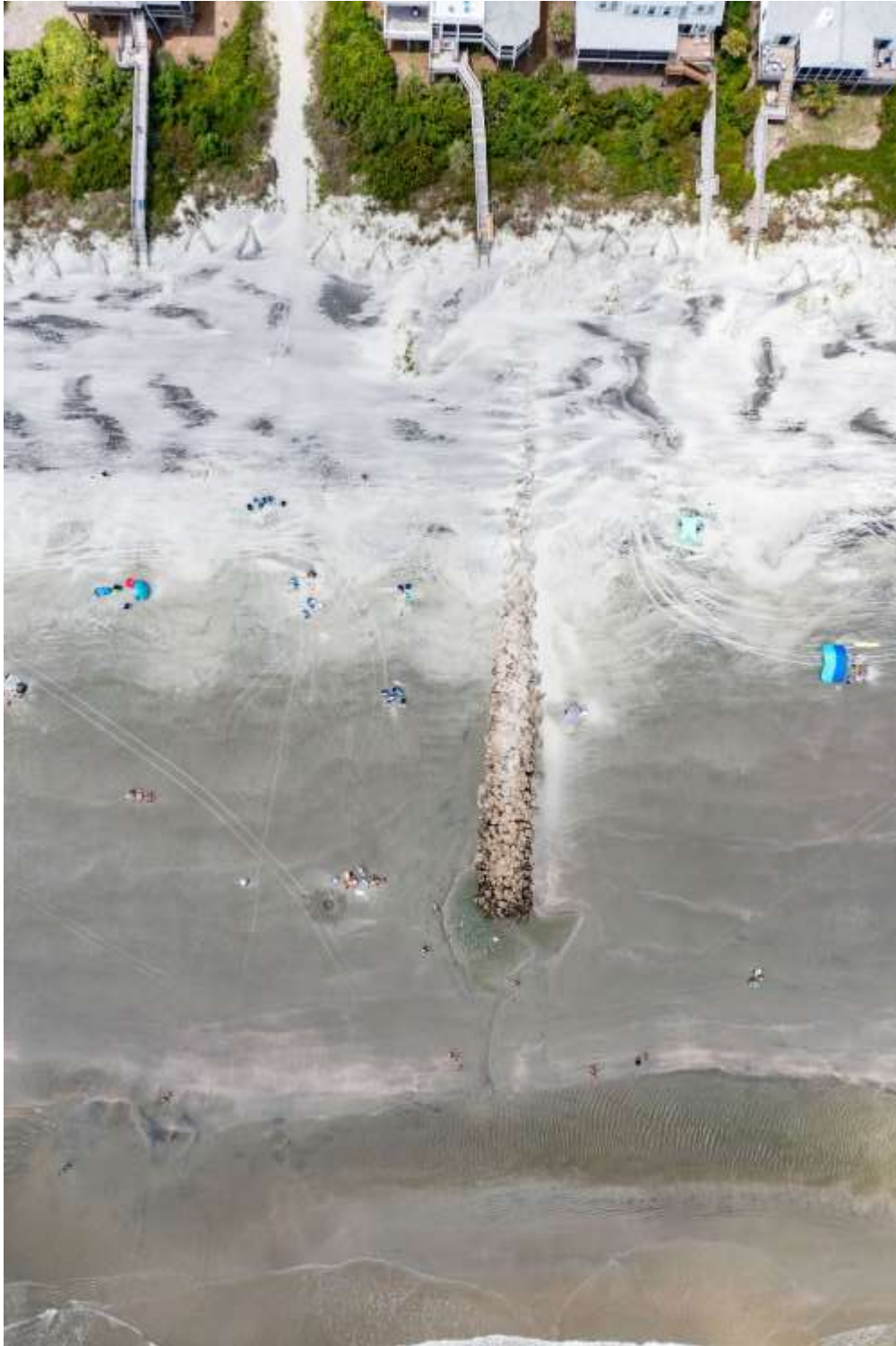
Figure 11. Groyne 28 in June 2021.
