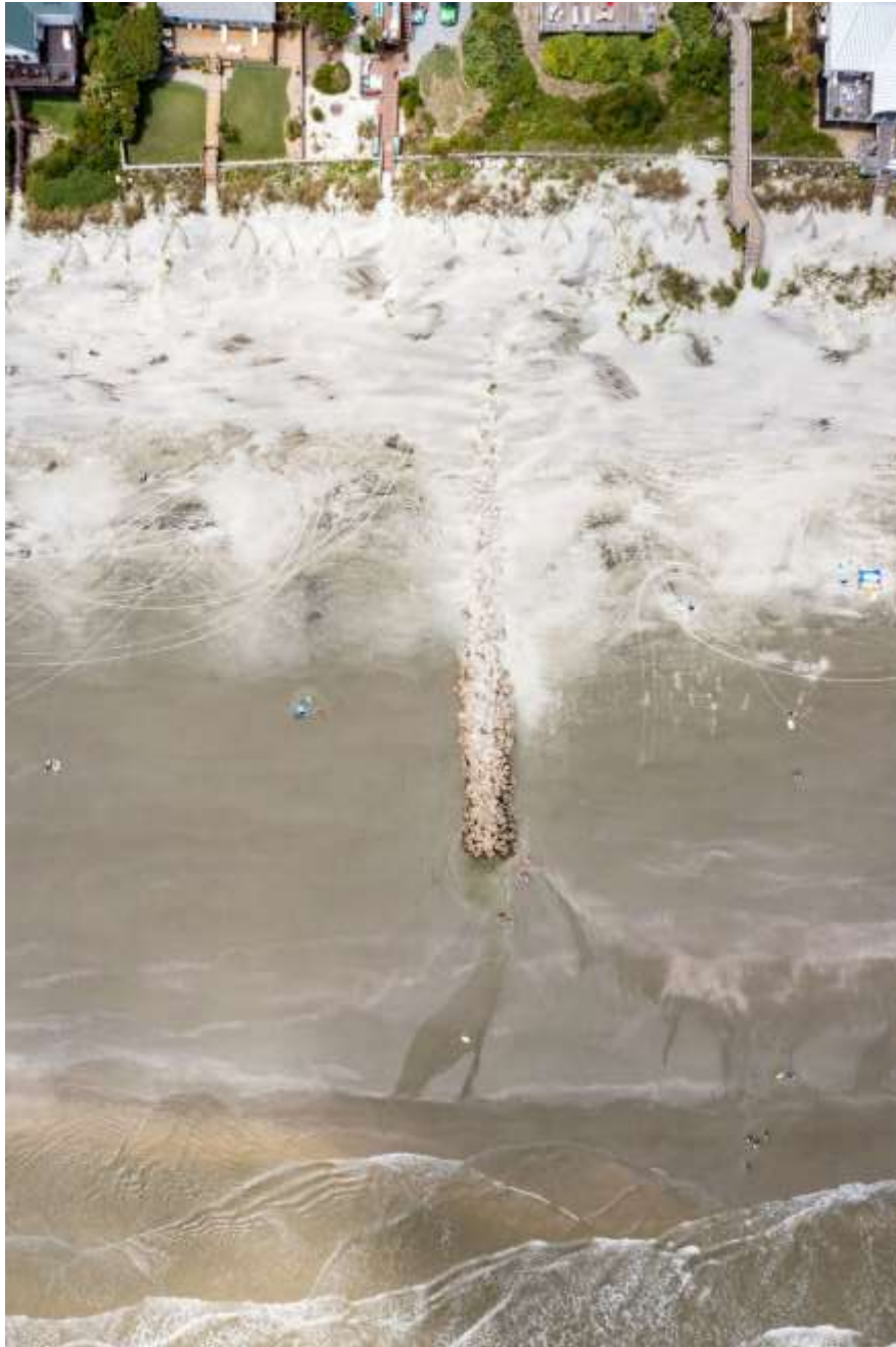
Figure 10. Groyne 27 in June 2021.
