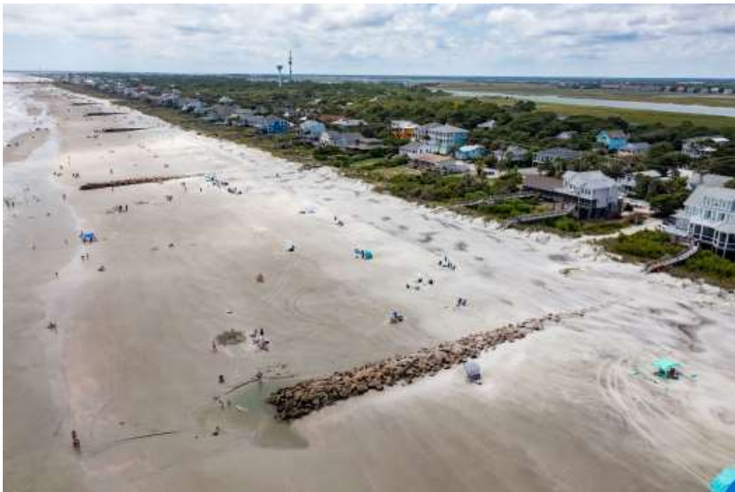
Figure 3. Oblique aerial photo of the west end of the rehabilitated groin field in June 2021 looking south at groins #28 and #29 (between 8th and 9th St. E.). The concrete cap groins that were rehabilitated by the Army Corps in 1993 are visible in the background east of the pier. No downdrift impacts were observed.
