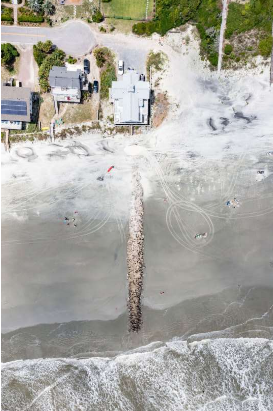
Figure 6. Groin 23 in June 2021.
