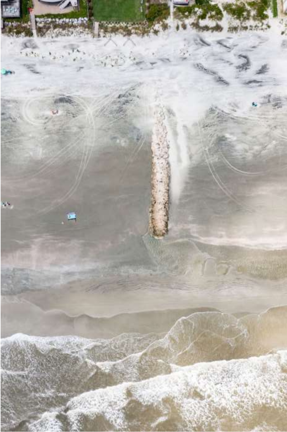
Figure 8. Groin 25 in June 2021.
