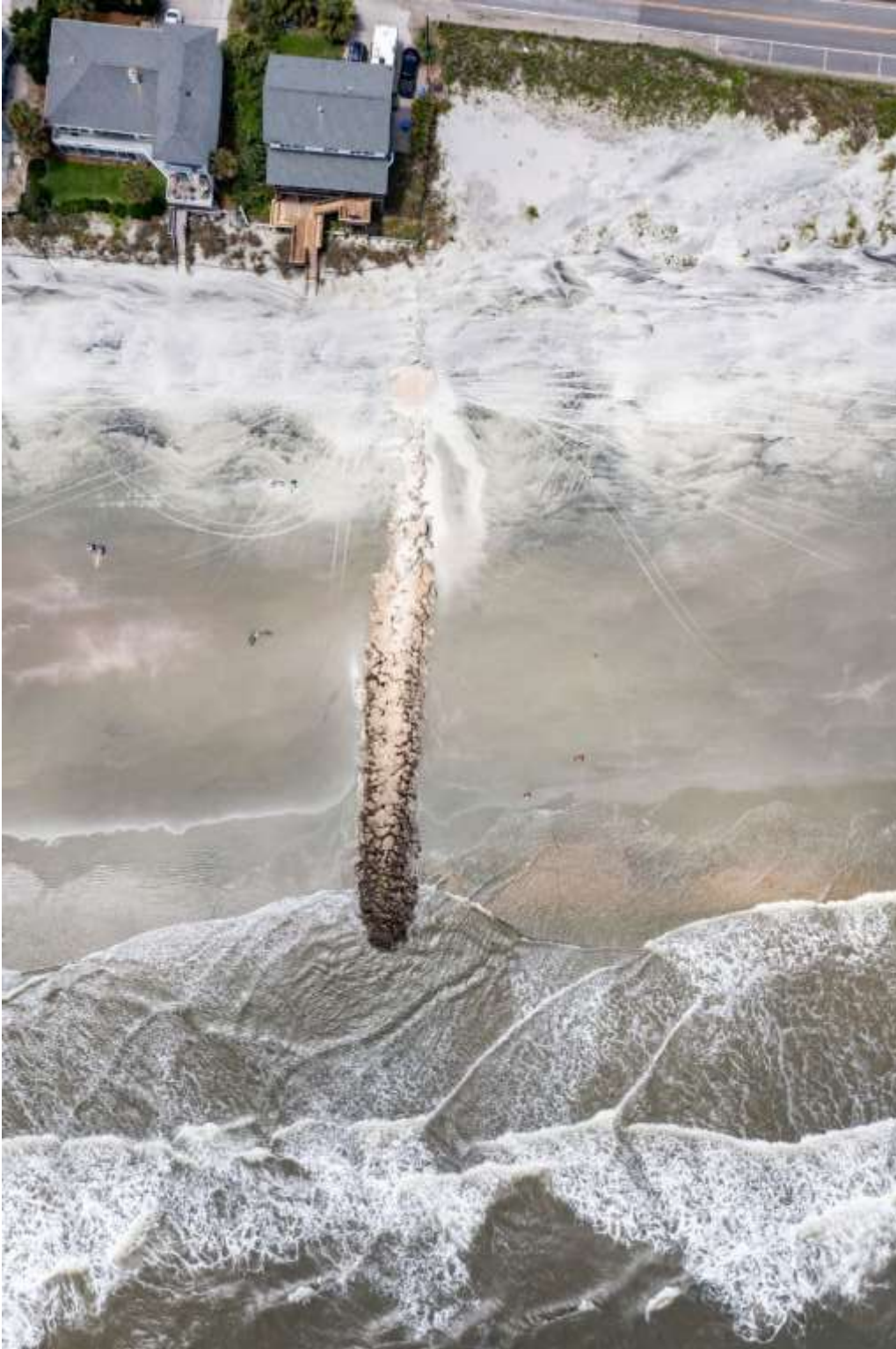
Figure 4. Groin 21 in June 2021 This groin is closest to the Washout by profile 2863.
