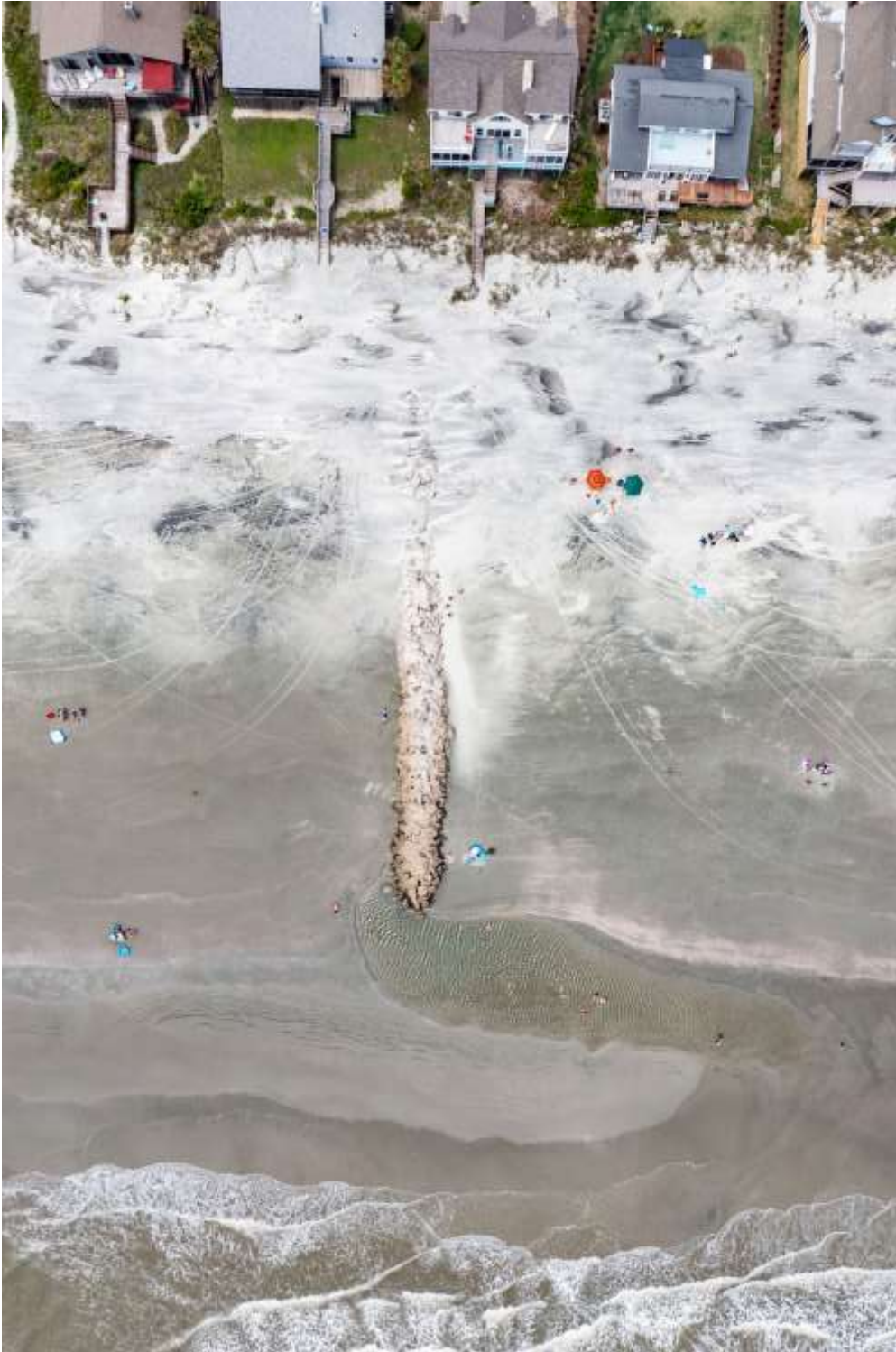
Figure 9. Groin 26 in June 2021.
