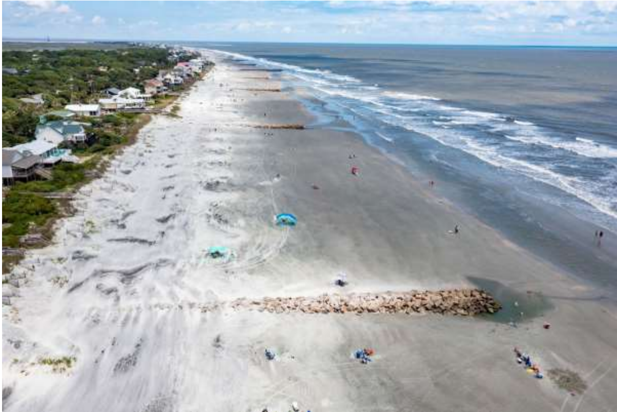
Figure 2. Aerial photo of the rehabilitated groin field in June 2021 looking northeast at groins #28 (near 9th St. E.) to #21 (near Washout). Note the advancing dune field, sand fencing and wide backbeach.
